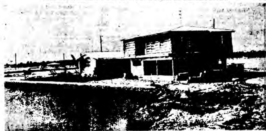
THIS IS CORAL POINT WHERE 128 HOMES WILL BE BUILT
