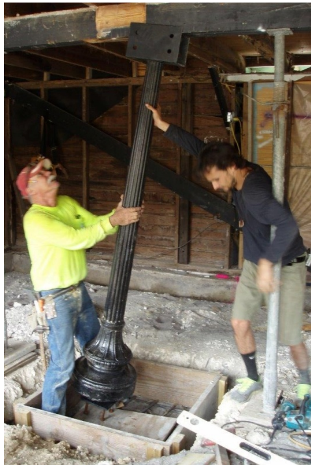
Ted Arpin and Son, Josh, reinstalling one of the lamp posts.
