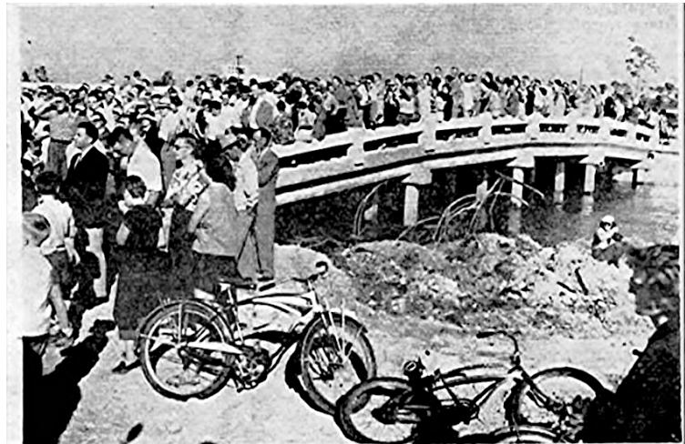
This is only part of the crowd of many hundreds jamming the new 26 Street-Galt Blvd. bridge over Middle River Sunday afternoon for the grand opening of the new span which now gives Wilton Manors a direct connection with Federal highway and a shorter route to the beach. Completion of the bridge is expected to quickly accelerate the already rapid development of this entire area.
