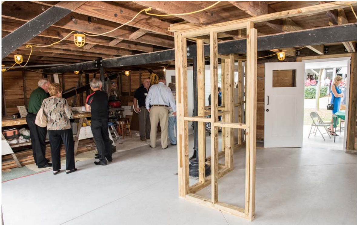
The Catering Preparation Area is framed in.
