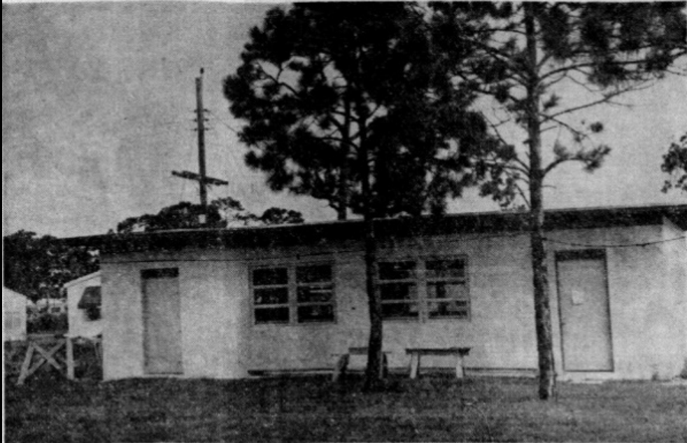
VILLAGE HALL — A tribute to the civic pride of rapidly growing Wilton Manors is the village hall, shown above. The building was constructed by the labor of the villagers, who spent their off time on Saturdays in working on the building. Wilton Manors is claimed by Mayor David Turner to be the fastest growing community in Broward county. At left is a new model home typical of those being built daily in the community.
