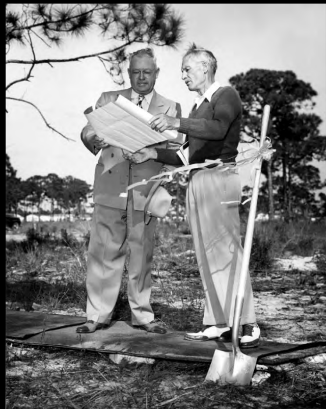
Turner (left) with Chairman of the Wilton Manors Civic Association, Norman Malcolm, at Village Hall groundbreaking)
