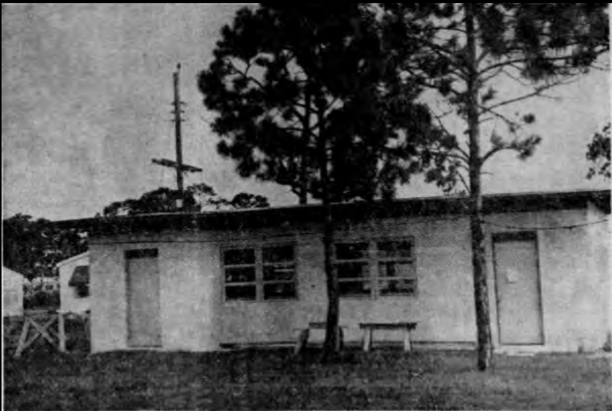
VILLAGE HALL — A tribute to the civic pride of rapidly growing Wilton Manors is the village hall, shown above. The building was constructed by the labor of the villagers, who spent their off time on Saturdays in working on the building. Wilton Manors is claimed by Mayor David Turner to be the fastest growing community in Broward county. At left is a new model home typical of those being built daily in the community.
