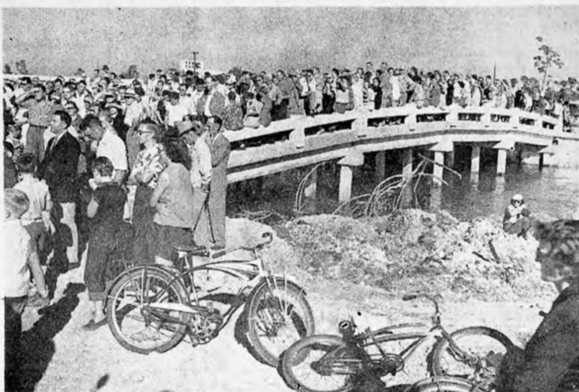
This is only part of the crowd of many hundreds jamming the new 26 Street-Galt Blvd. bridge over Middle River Sunday afternoon for the grand opening of the new span which now gives Wilton Manors a direct connection with Federal highway and a shorter route to the beach. Completion of the bridge is expected to quickly accelerate the already rapid development of this entire area.
