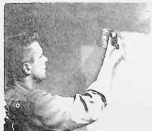
Start with the ceiling and paint across the narrow dimensions.
