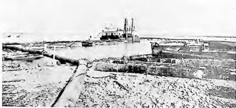
Port Everglades dredged to 35-foot depth
