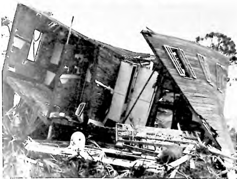
Wreckage left by hurricane (KELCY PHOTO)
