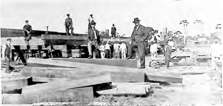
Governor N. B. Broward inspects construction of dredge "Okeechobee" (GIFT, W. T. KENNEDY)
