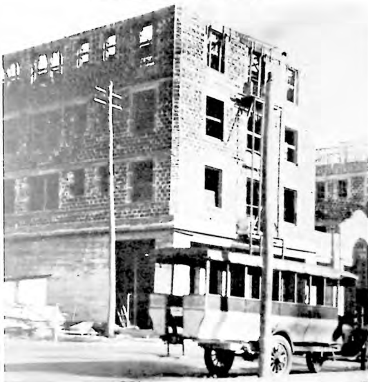
Hotel Broward under construction (VAH. COLLECTION)
