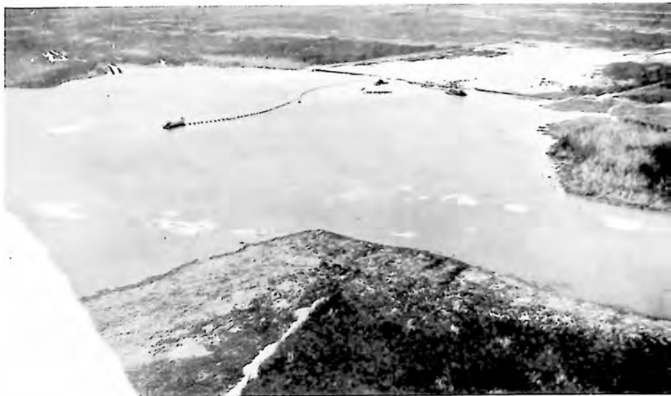
(KELCY PHOTO) Dredging of Port Everglades at Lake Mabel
