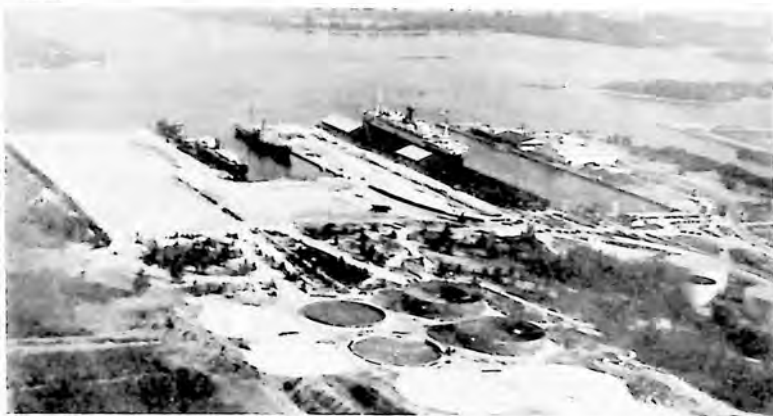
Below: Tank farms under construction at Port Everglades (BURGHARD COLLECTION)
