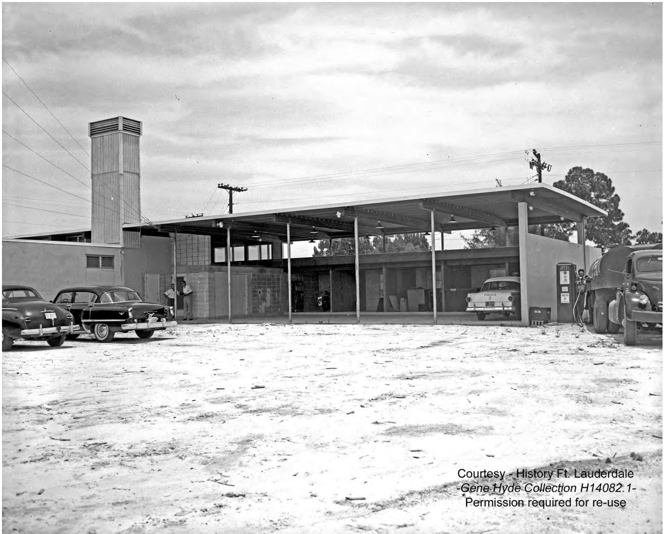
1957 new City Hall nearing completion, rear service area
